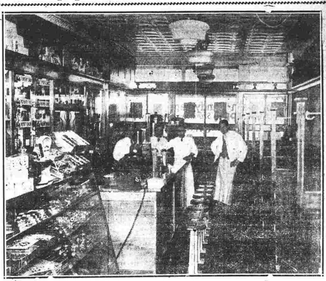
Wachtel's Department store at Nos. 376-392 Front street has installed a new fountain, candy department and luncheonette service, which opened on Thursday with a large crowd taking advantage of the improved facilities.
